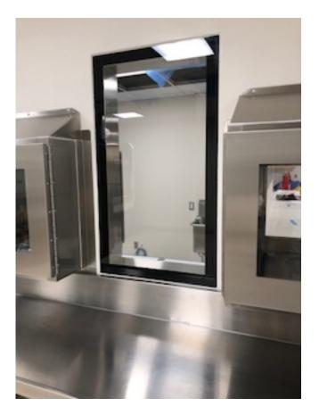
Cleanroom Window Borderless Flush mount (cleanroom side) Glass panel
